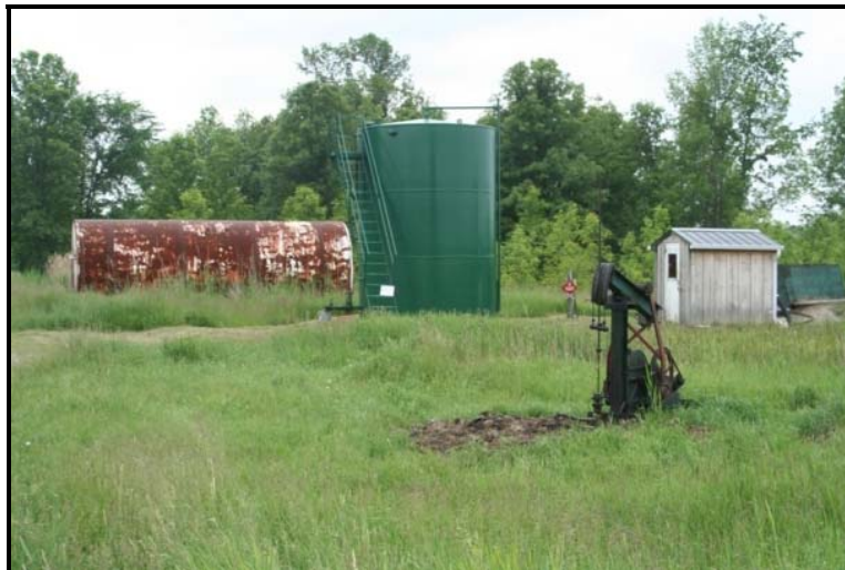
Figure B-23: Receiving tanks on South Byers field.
