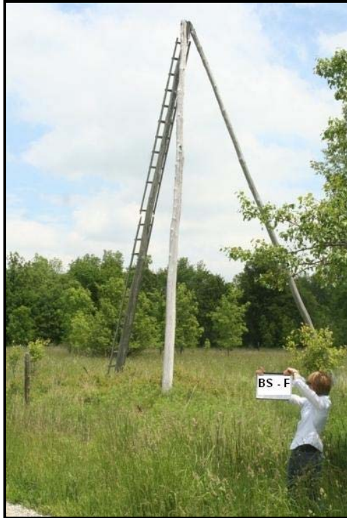
Figure B-24: Feature BS-F, last standing original three-pole derrick in the Oil Springs oil field. (located in the South Byers Field)
