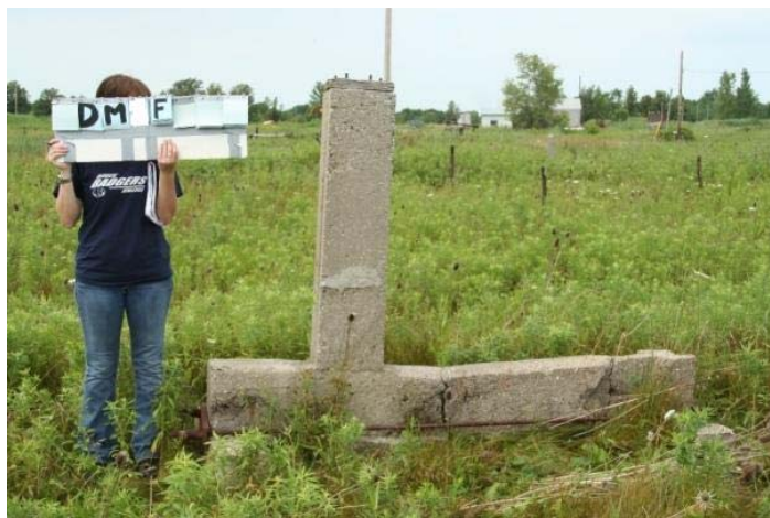
Figure C-4 Experimental concrete jerker line post
