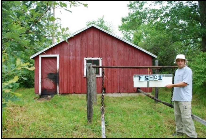
Figure B-3: Powerhouse FS-D1, South Fairbank Field
