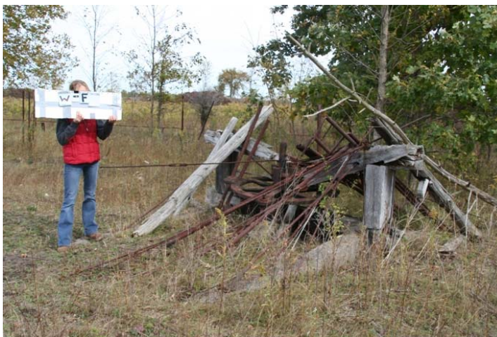
Figure C-7: Cast iron field wheel with collapsed timber frame in Woods Field.
