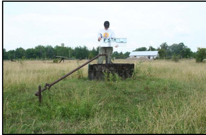
Figure B-18: Feature FS-X, small in-ground day tank on Fairbank Property, with old piping still attached
