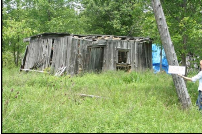
Figure C-9: Abandoned-in-place power house on the Byers South Field
