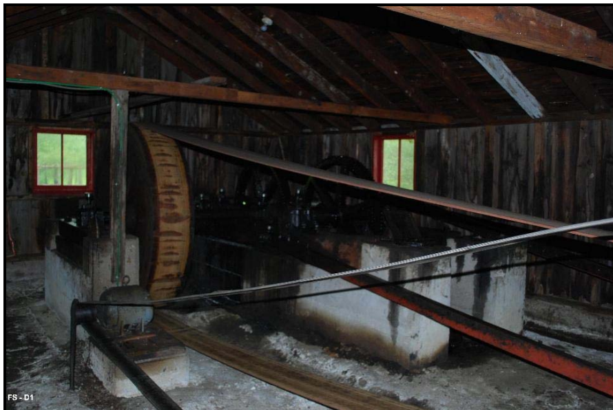
Figure B-4: Interior of Powerhouse FS-D1, South Fairbank Field
