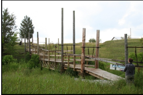
Figure B-31: Bridge for maintenance crews to inspect jerker line over Black Creek on Fairbank Field.
