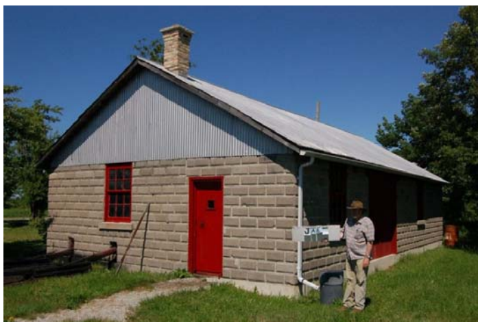
Figure C-5: Concrete block enginehouse on the James Field
