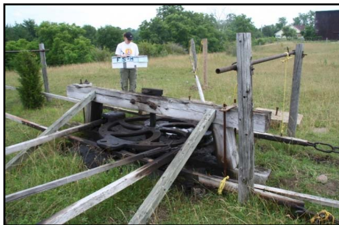
Figure B-6: Bull wheel at Orchard Rig (FS-M) with connecting roads leading from powerhouse on left side. A double field line runs diagonally from upper left to lower right while a single line extends to the centre/back of the photo
