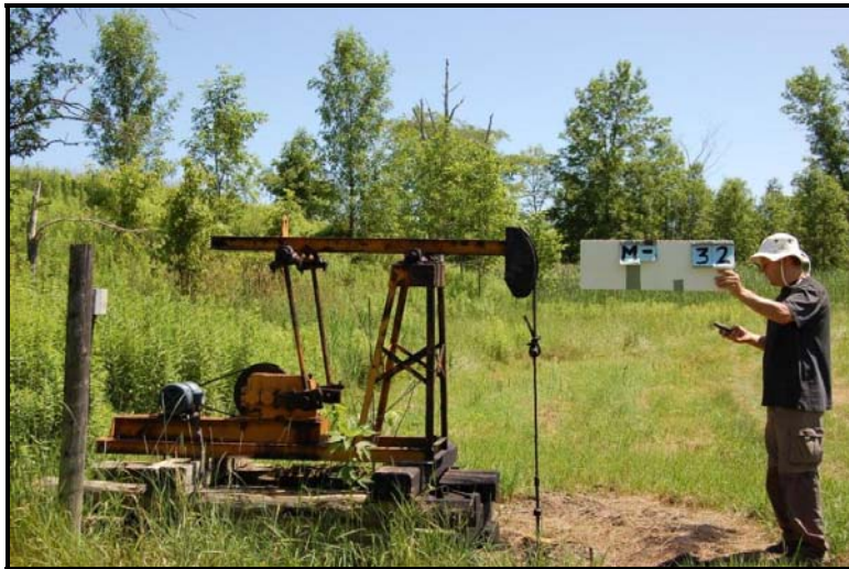
Figure B-17: Feature M-32, individually powered steel well on the Morningstar Property
