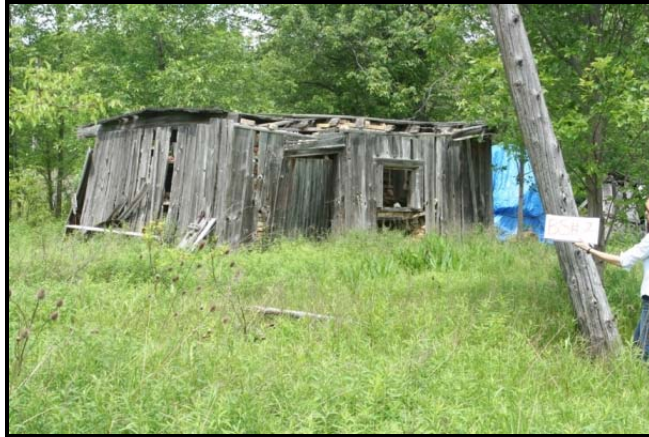
Figure B-5: Power house BS-B on the Byers South Field
