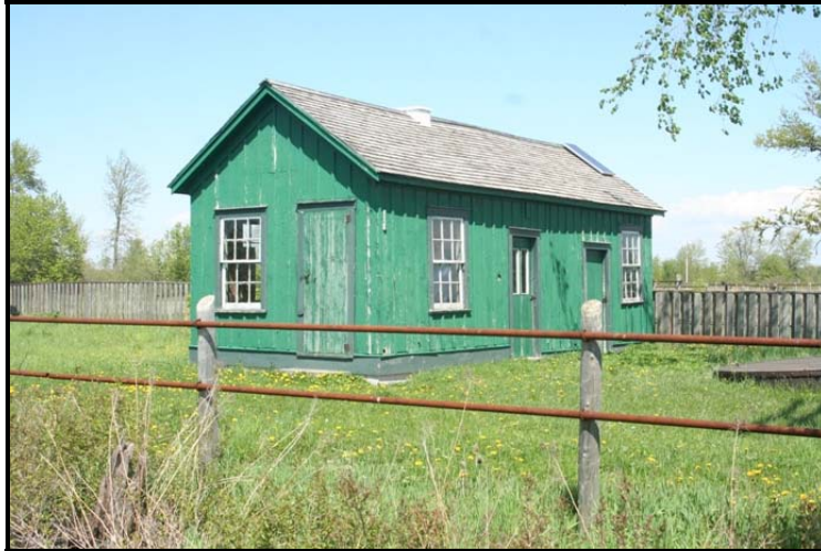
Figure B-22: Pump room at former receiving station at Kelley Road and Gum Bed Line
